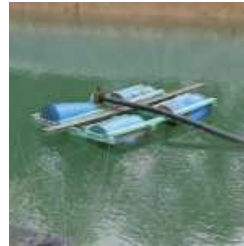
Water recycling system
